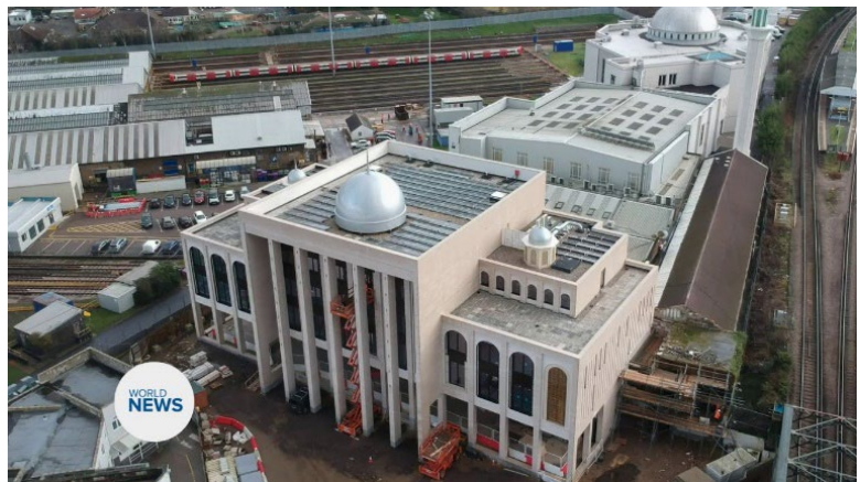
Figure: Solar panels on top of Bait-ul-Futuh Mosque
